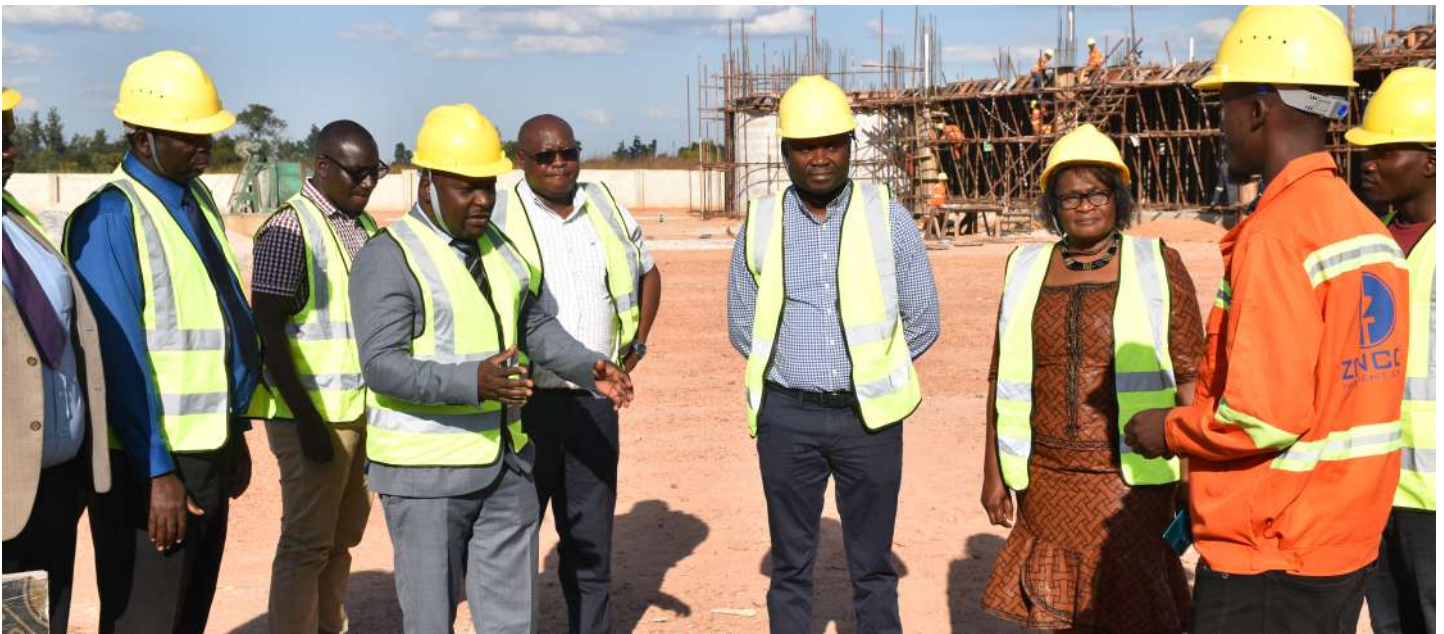
ZABS Board Chairperson Mr. Mbope Nyondo along side other Board members and ZABS management during a tour of the Laboratories being constructed off Airport Road
